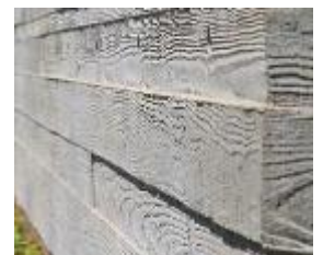
adze texture concrete
