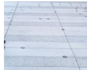
horizontal scored concrete
