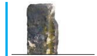
Lake Washington Boulevard system • Stone transition features
