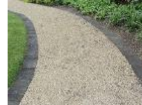
gravel pathway with concrete edging
