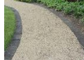
gravel pathway with concrete edging
