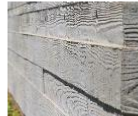
adze texture con- crete wall
