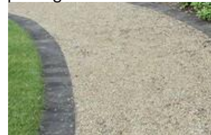
gravel edged with concrete
