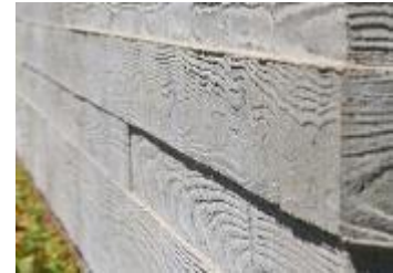
adze texture concrete seating walls
