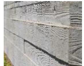
adze texture concrete
