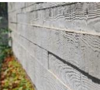
adze texture concrete walls
