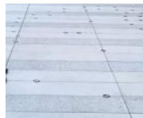
horizontal scored concrete
