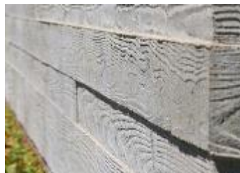
adze texture concrete site walls
